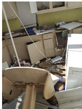
Inside one of the classroom areas.
